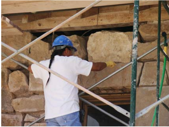
Tommy prepares the voids to be repointed.
