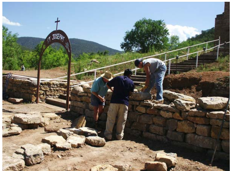
Learning the art of dry stone wall construction from master waller Pete Mold are Walter Scott, Brother Peter and Christian Aldava
