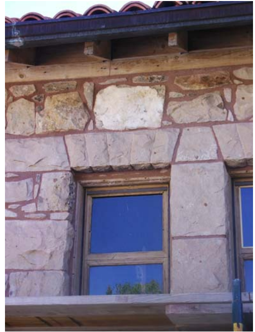
View of finished wall
