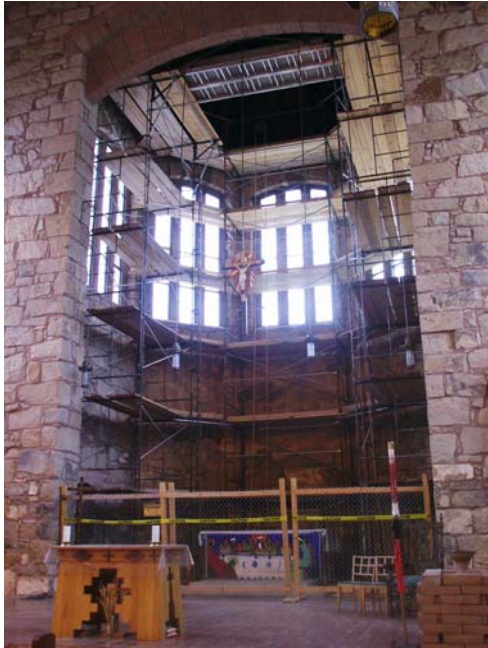
The apse with scaffold, ready for restoration.
