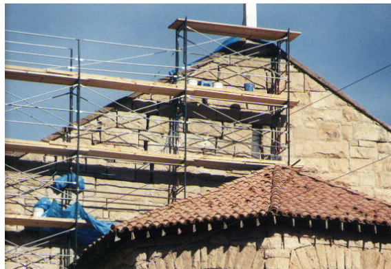
Examples of the stonework after deteriorated mortar is removed.
