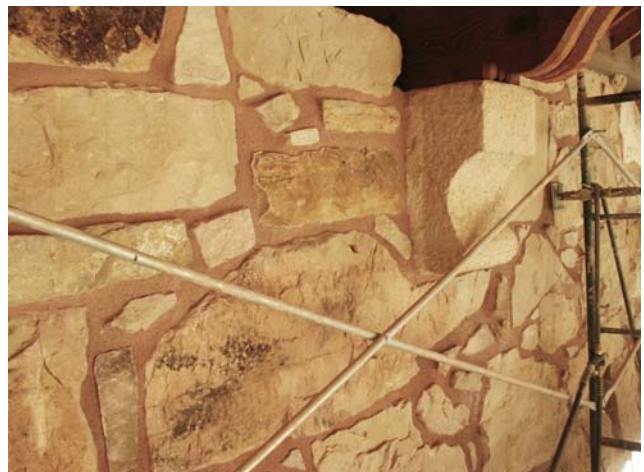
Here is a demonstration of “Before” and “After” our repointing work at the top of the north wall interior.
