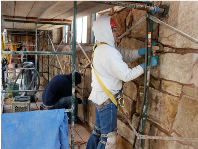
The Restoration Crew repointing the stonework of the north wall interior.
