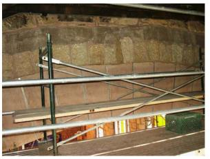
Besides repointing the stonework above the arch, the sheet metal and stucco cover that hides the steel I-beam arch support is limewashed to match the color of the mortar.
