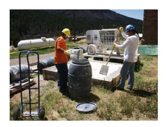
Restoration-trainee Walter and Tommy bring in the newly prepared lime putty for the mortar. The hydrated lime is being donated by the Chemical Lime Company.
