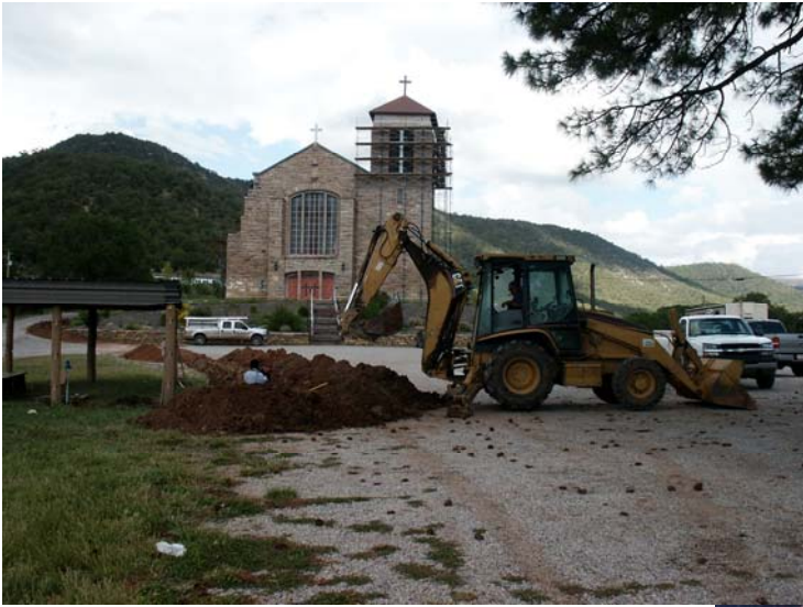
Tribal Water Department putting in new waterline.
