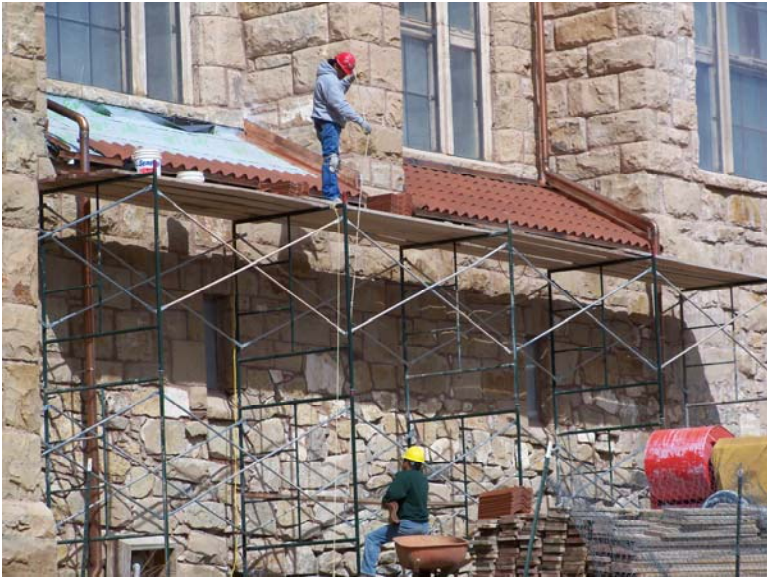
Tommy & Martin working on alcove roof
