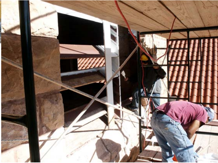
Martin & Sam working on Belfry louvers.
