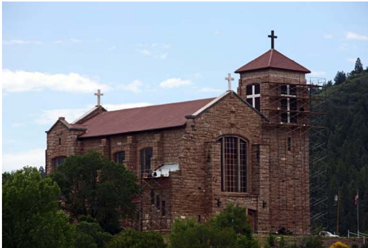
The crew working on Choir loft stair case roof.
