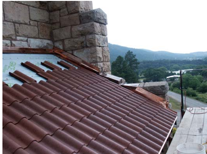
Roof almost completed.
