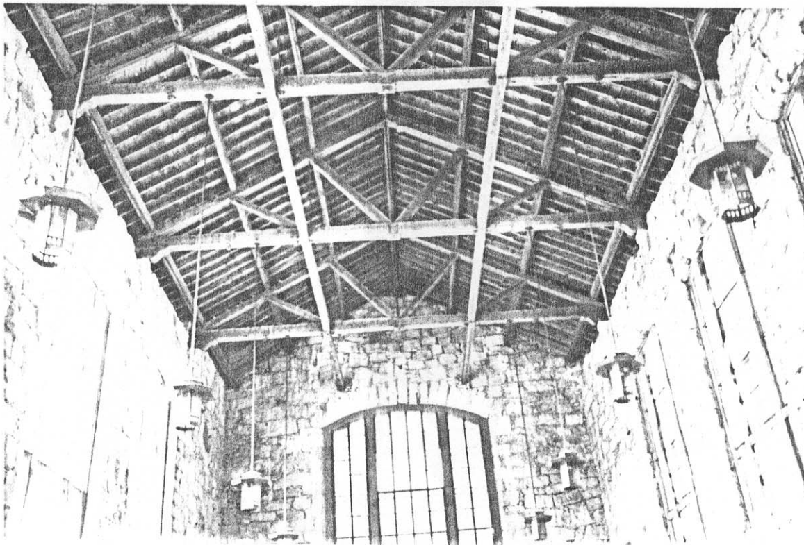
Figure 10: Interior roof support system
