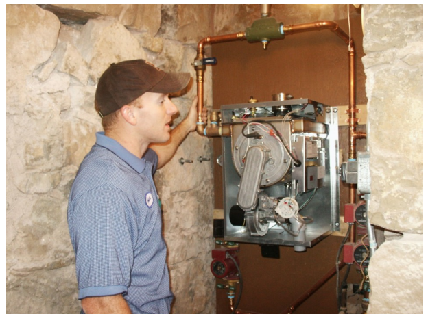
Josiah installing the new boiler.
