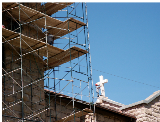
Tommy painting the cross while the crew works on belfry
