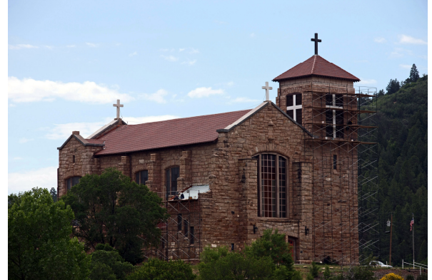
Martin & Sam working on Choir loft roof.
