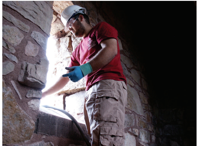
Trainee David Walters working on a alcove window .
