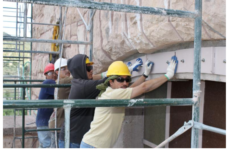
Ethan & Gilbert working with crew on west window.
