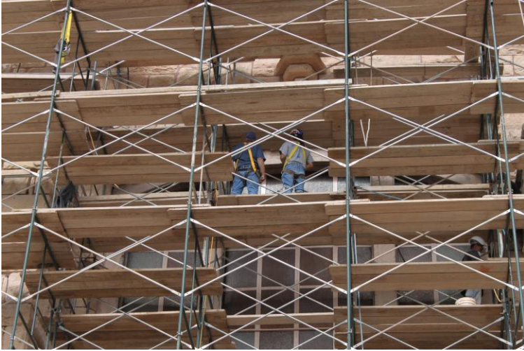
Carroll & Tommy inspecting the arch.
