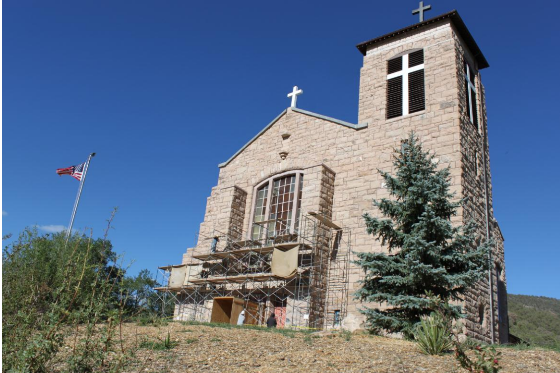
The crew & trainees removing the scaffolding for the summer.
